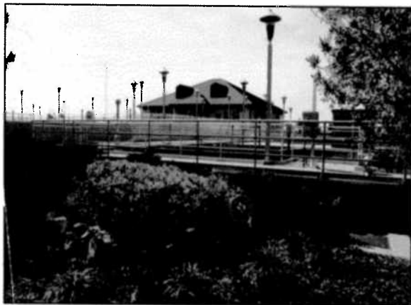
Thomas E. Taylor Water Treatment Plant - Lewisville, TX
